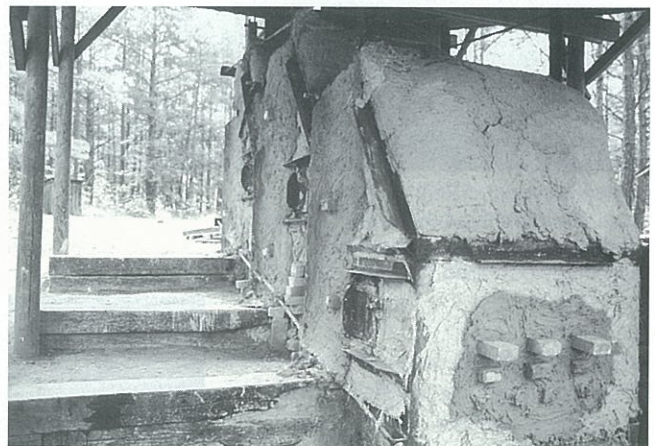
Metal framework braces the walls and arches of the Bruhins' three-chambered climbing kiln.
